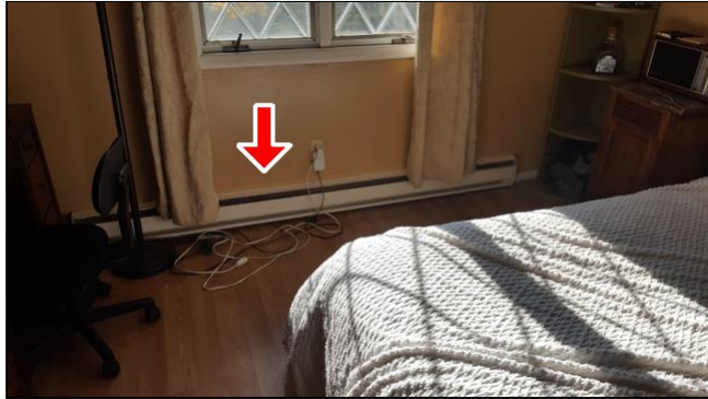
7.0 Item 1(Picture) Baseboard heater not operational
