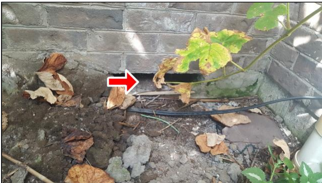
2.3 Item 1(Picture) Missing block at foundation
