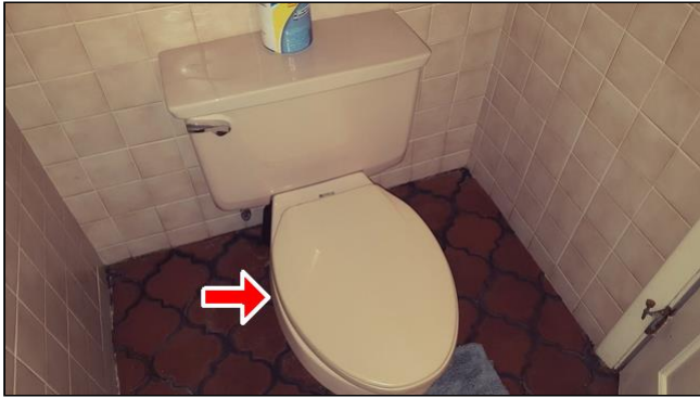
5.1 Item 2(Picture) Loose and leaks
