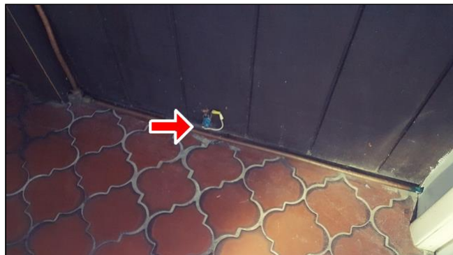
6.3 Item 4(Picture) Exposed wires
