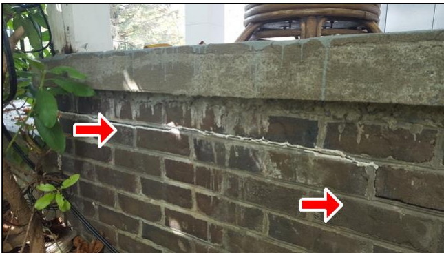
2.3 Item 3(Picture) Cracked brick joint at porch
