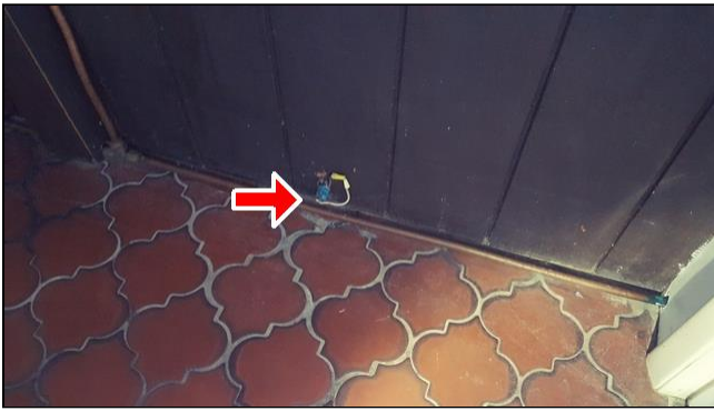
6.3 Item 4(Picture) Exposed wires
