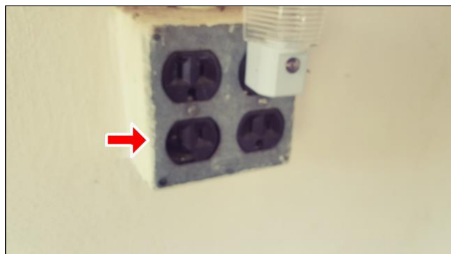
6.3 Item 2(Picture) Broken outlet
