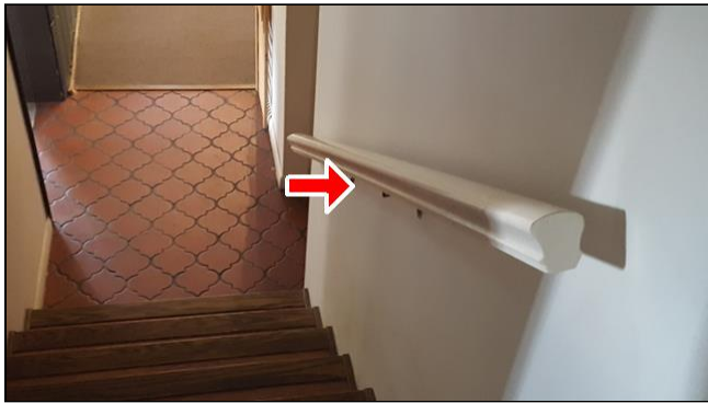
3.3 Item 1(Picture) Loose handrail
