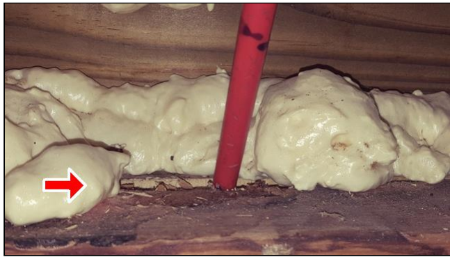
4.3 Item 1(Picture) Rotted sill plate
