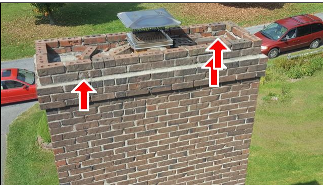
1.2 Item 1(Picture) Deteriorated mortar and loose bricks
