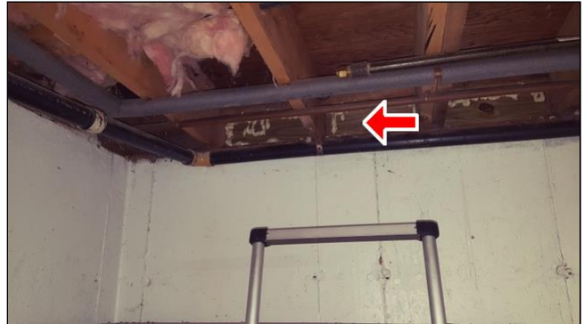
4.3 Item 4(Picture) Water damage and WDI damage
