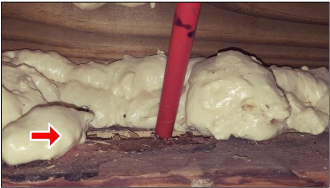
4.3 Item 1(Picture) Rotted sill plate
