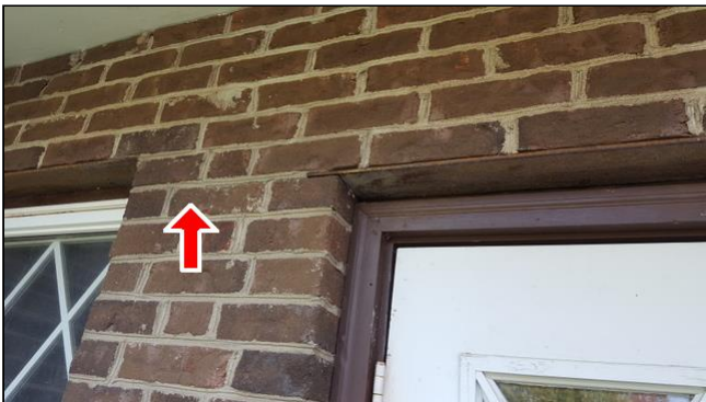
2.0 Item 4(Picture) Mortar cracking
