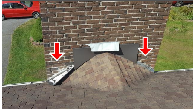
1.1 Item 2(Picture) Missing counter flashing
