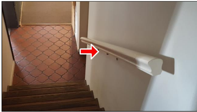
3.3 Item 1(Picture) Loose handrail
