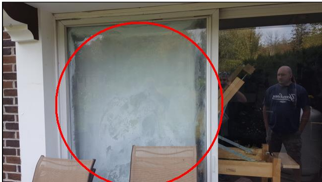
2.1 Item 1(Picture) Broken thermal seal
