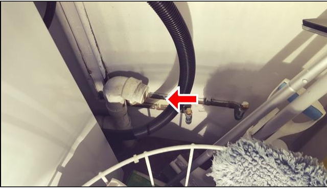
5.0 Item 1(Picture) Open drain line
