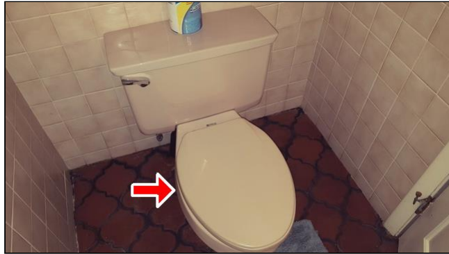
5.1 Item 2(Picture) Loose and leaks
