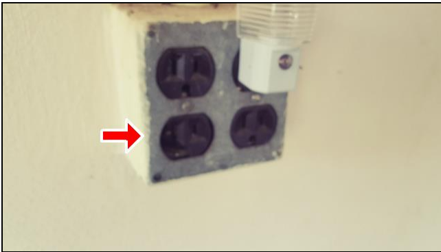
6.3 Item 2(Picture) Broken outlet
