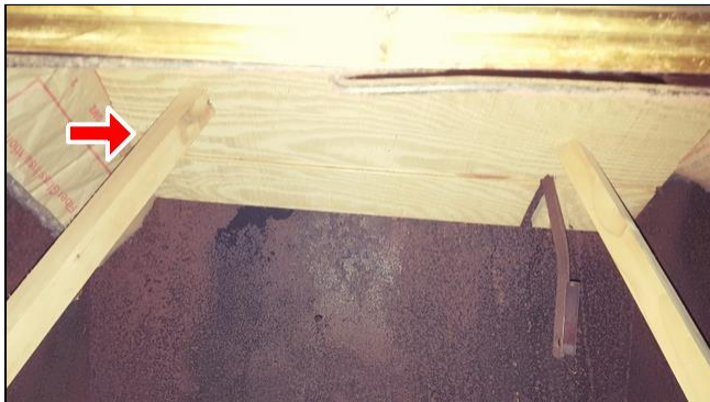
7.6 Item 2(Picture) Flue blocked
