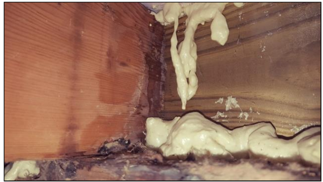
4.3 Item 2(Picture) Rotted joist and sill plate
