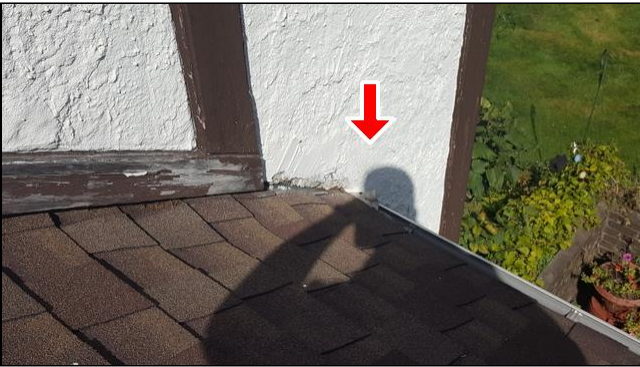
1.1 Item 3(Picture) Kick out flashing recommended
