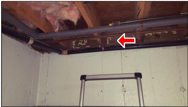
4.3 Item 4(Picture) Water damage and WDI damage
