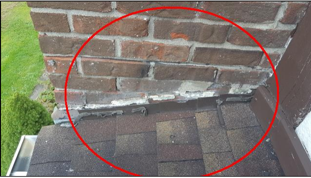
1.1 Item 1(Picture) Missing counter flashing
