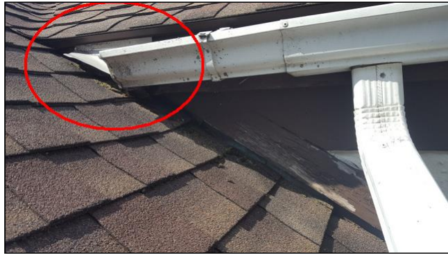
1.1 Item 4(Picture) Flashing repairs needed
