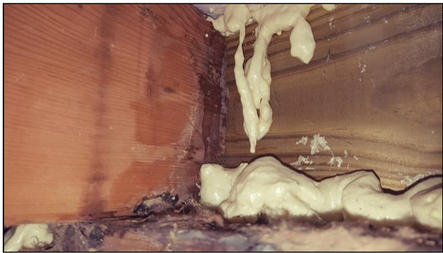
4.3 Item 2(Picture) Rotted joist and sill plate
